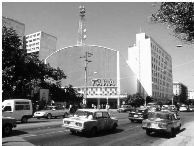
The 1947 Radiocentro building displays a curved marquee that takes its form from the street corner at L Street before re-emerging on the La Rampa side as a thin-shell undulating canopy with a projecting horizontal beam fixed at one end (what we architects call “cantilevered”) that defines the first floor retail spaces.
