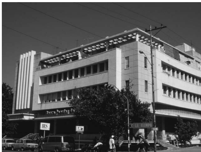
The Viguma Real Estate Co. building, a mixed-use apartment and retail structure, is raised on pilotis , in the style of Le Corbusier, that break through at the upper floor to visibly support the concrete canopy covering the roof deck. At the sidewalk the façade sets back to expose a lower and upper retail floor.
