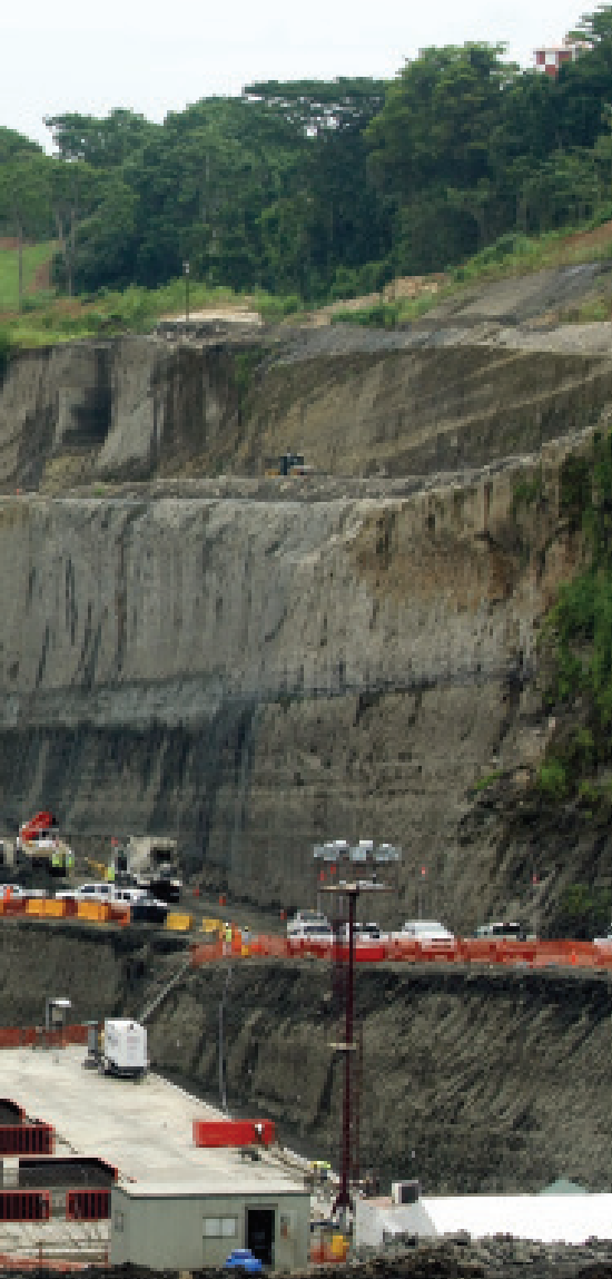
Left: The third set of locks is shown under construction in Gatún. Concrete is being poured for the foundation of the third set of locks in the Atlantic area in preparation of the excavation and removal of a large quantity of dirt. The photo was taken on June 1, 2011. Above: Panama Canal workers (ACP) perform maintenance on the Miraflores locks on September 6, 2011.
